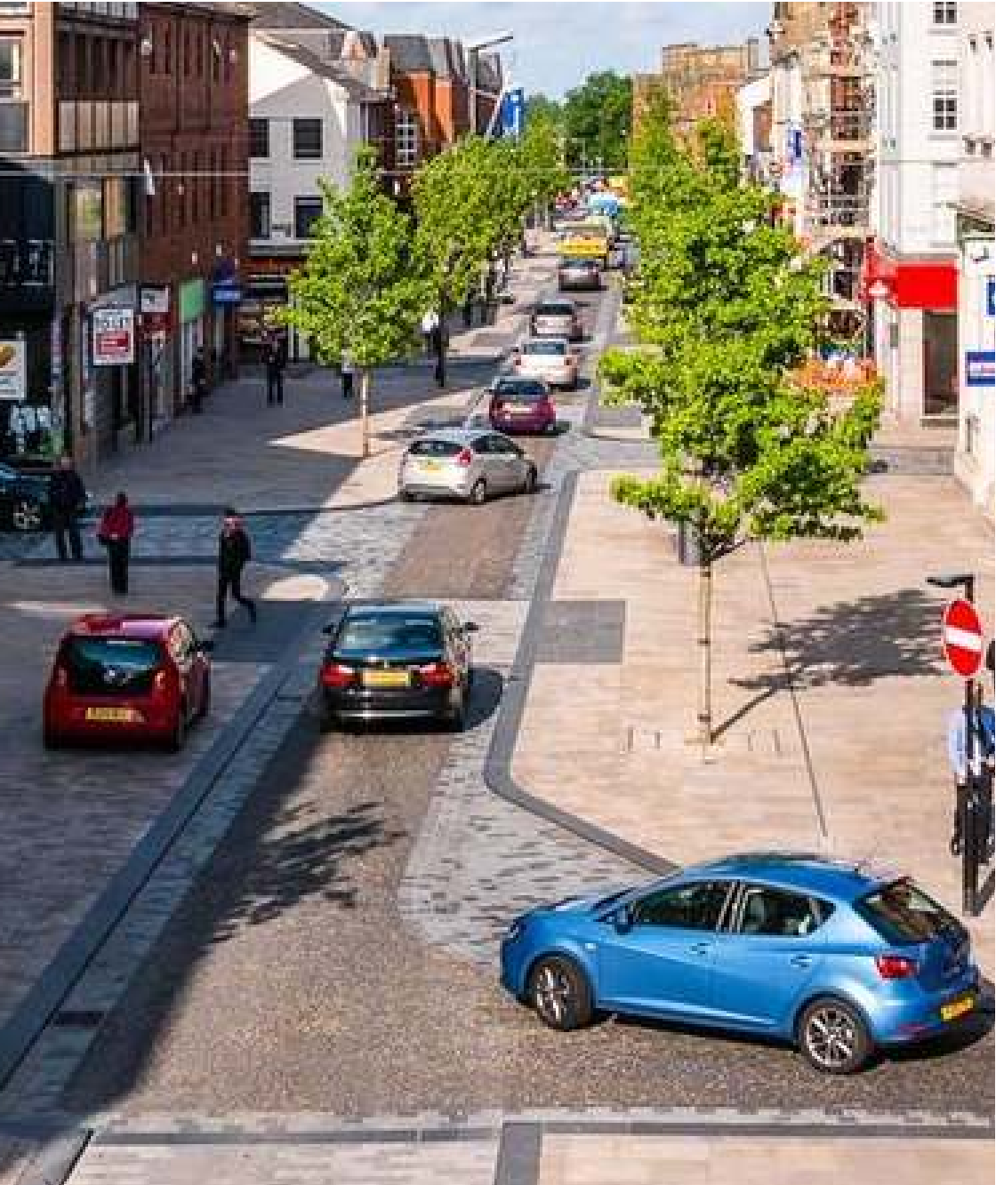
Gambar 18 Shared street di Lancashire Country Council Sumber : planetradio.uk
