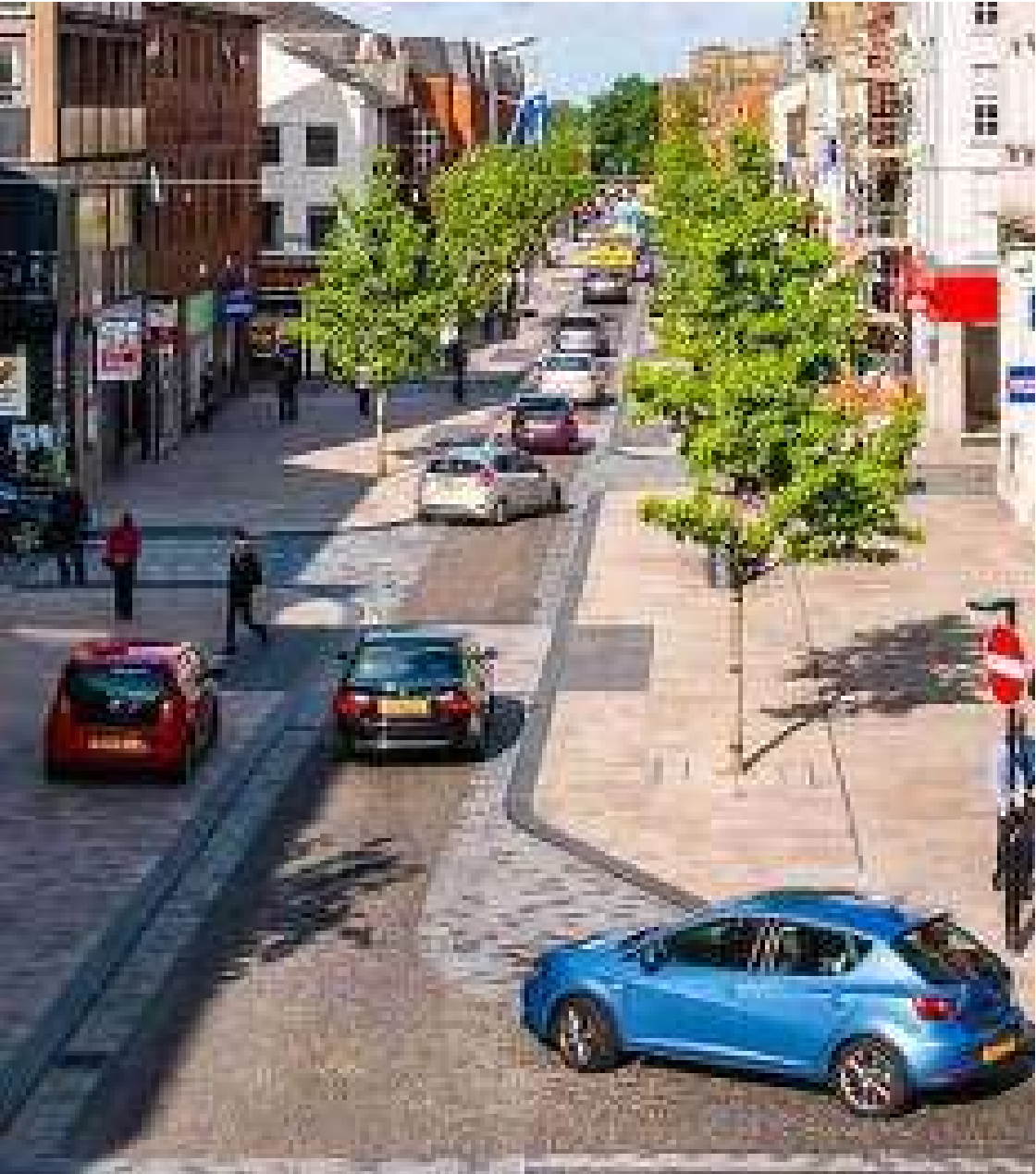
Gambar 18 Shared street di Lancashire Country Council Sumber : planetradio.uk
