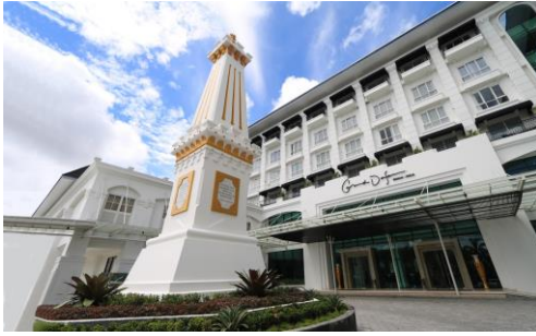
Gambar 3. 1 Gedung Hotel Grand Dafam Rohan Jogja
